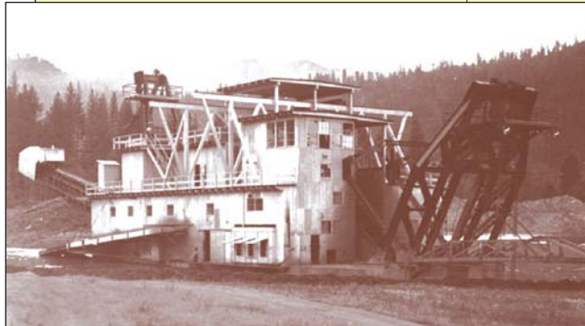
Gold mining dredge, Junction City district, Trinity River, 1935. Note the bucket line behind the gantry at the near end (right side) of the dredge, the stacker conveyor discharging coarse tailings at the far end, and the side sluice discharging fine tailings to the rear. The dredge separated the coarse material in a rotating trommel inside the housing, and fine material passed through sluices and over tables charged with mercury to capture the gold. Gold dredging occurred on more than a dozen Sacramento and San Joaquin river tributaries between 1898 and 1968, distributing mercury into the river system (see p.2).
