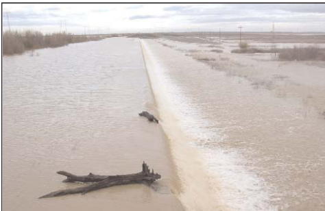
Raising the height of this outlet weir is one of a number of possible improvements to a 1930s-era settling basin where Cache Creek empties into the Yolo Bypass near the city of Woodland. The basin traps an estimated half of the mercury coming downstream in wet years.
